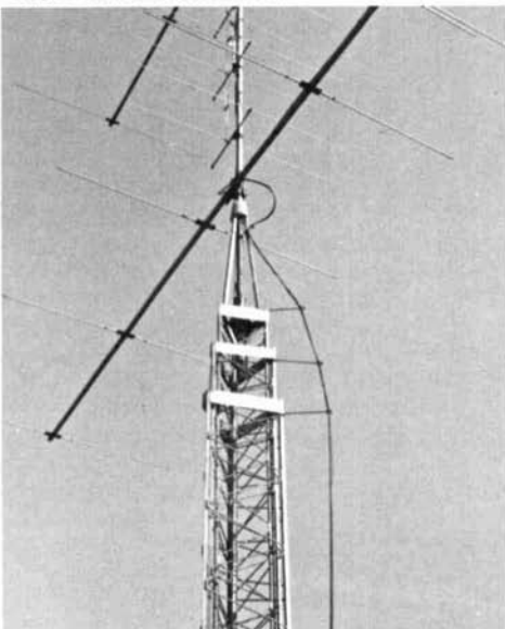
Top of tower construction.
